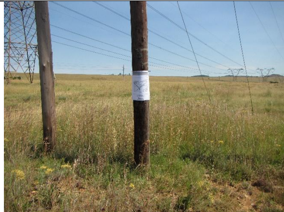
Proposed Siyathemba switching station and powerline site
