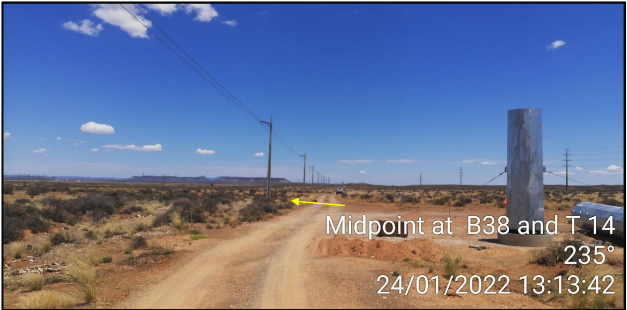
Photograph 2: illustrating the middle point of the 4.5km Bypass powerline together with the surrounding infrastructure and surrounding environment.
